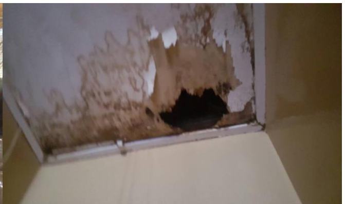
Part of the linking ceiling
