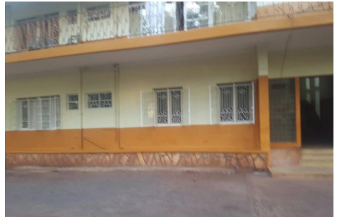
New front side of Rubaga Students Centre after renovation
